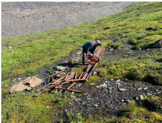
PHOTO 3 – NEBCWF crew cutting pipes for easier transport. Photo: T. Fulton, August 2022.
