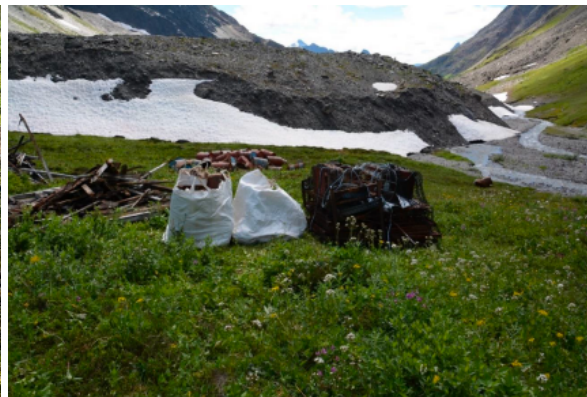
PHOTO 4 – Sorted waste ready for transport and disposal. Metal waste (R) is netted for helicopter slinging. Photo: T. Fulton, August 2022.
